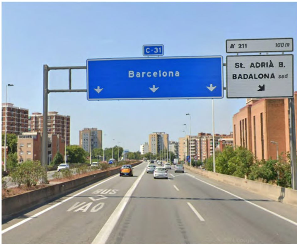
Figure 16: Dedicated bus and carpooling lane on the C-31 in Barcelona © Google Street View (2021)
